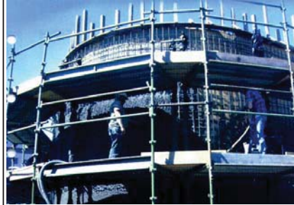
Fig 1b - Water tanks 20m diameter and 5m tall have been constructed in one day with silica fume shotcrete. An internal shutter about 3m long and full height is moved like a horizontal jump form.
