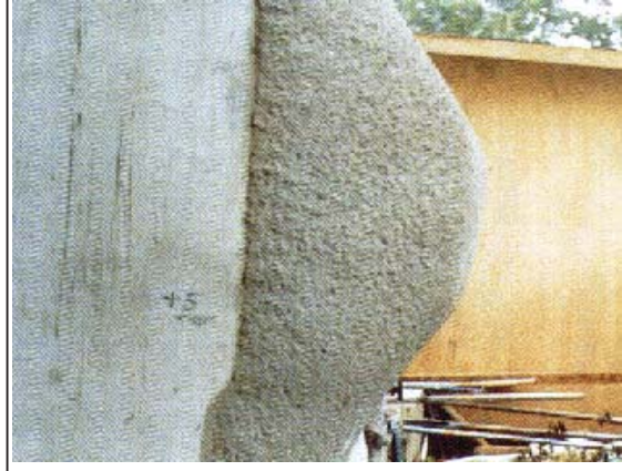
Fig 8 – Silica fume shotcrete can be built up to 10x that of normal shotcrete
